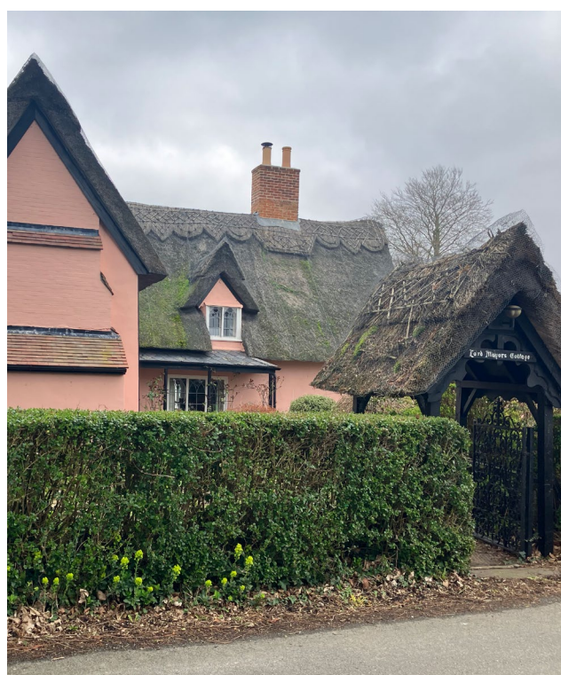
Figure 22: Historic thatched cottage with tall chimney stacks.
