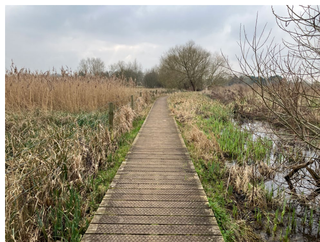
Figure 38: Man made timber and chicken wire footpath alongside the nature reserve providing access to Mildenhall and River Lark.
