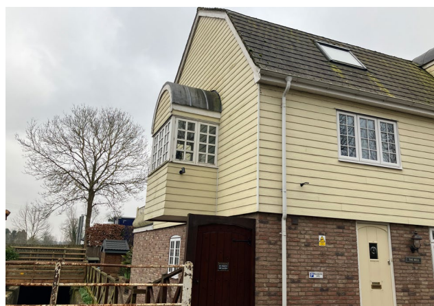
Figure 25: The Mill, which has been retrofitted with yellow painted timber panels.
