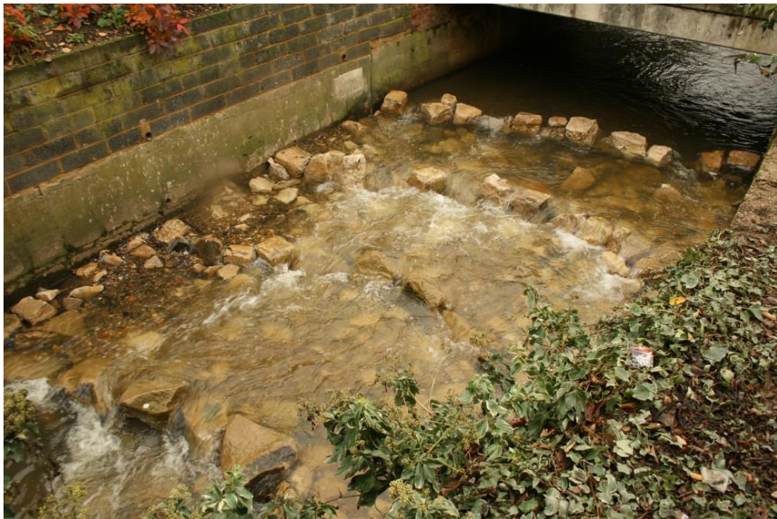
Fig 10. Rock ramp, the bed is lowered and replaced with designed boulder placement, the cross section of the channel is increased improving flood discharge.
